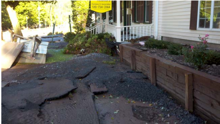
Damage to right driveway
